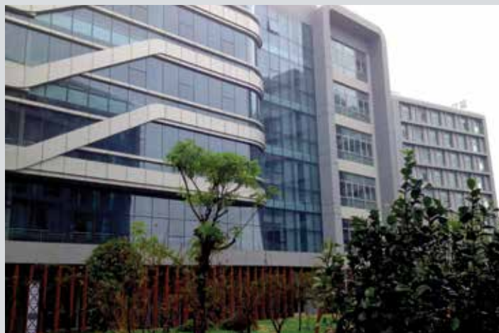
Stepan's new Nanjing, China R&D facility - top floor
