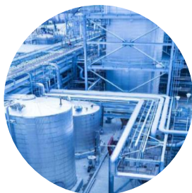
Stepan Fermentation Plant Lake Providence, LA
