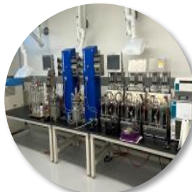
Fermentation Lab Installation Global Technology Center
