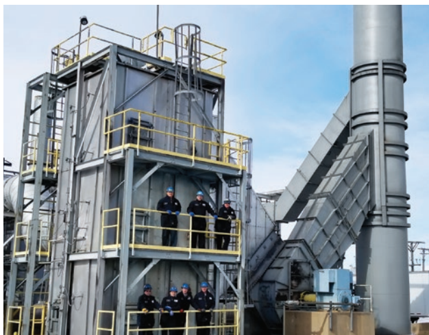
NEW CATALYST TECHNOLOGY REDUCED PHTHALIC ANHYDRIDE COMBUSTOR EMISSIONS BY 66% AT OUR MILLSDALE, IL, FACILITY.
