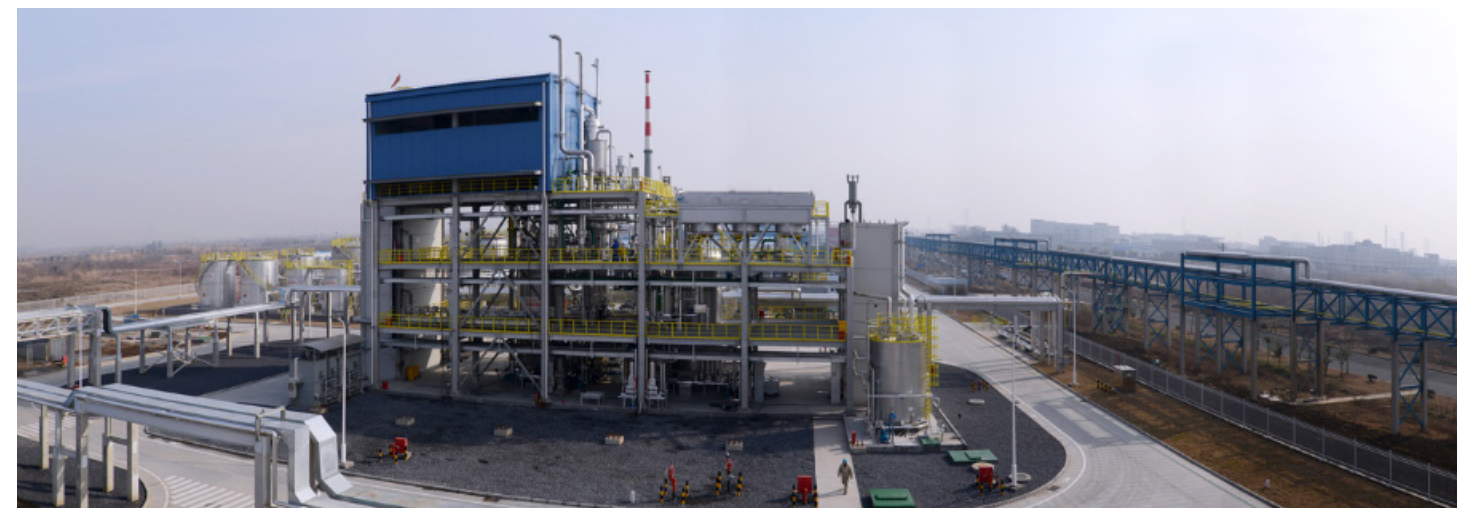
Stepan's Manufacturing Facility in Nanjing, China
