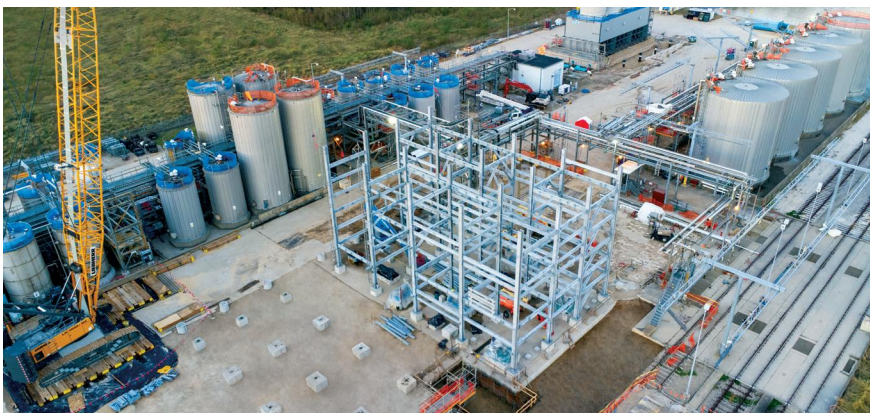
Construction in Progress: Alkoxylation Plant, Pasadena, Texas
