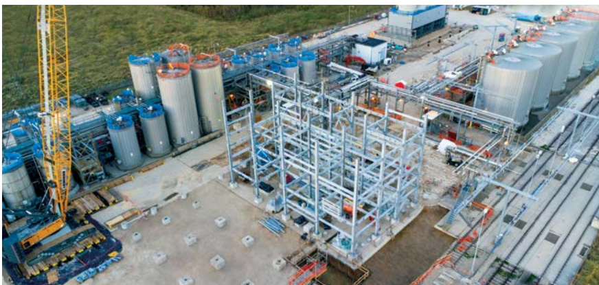
Construction in Progress: Alkoxylation Plant, Pasadena, Texas
